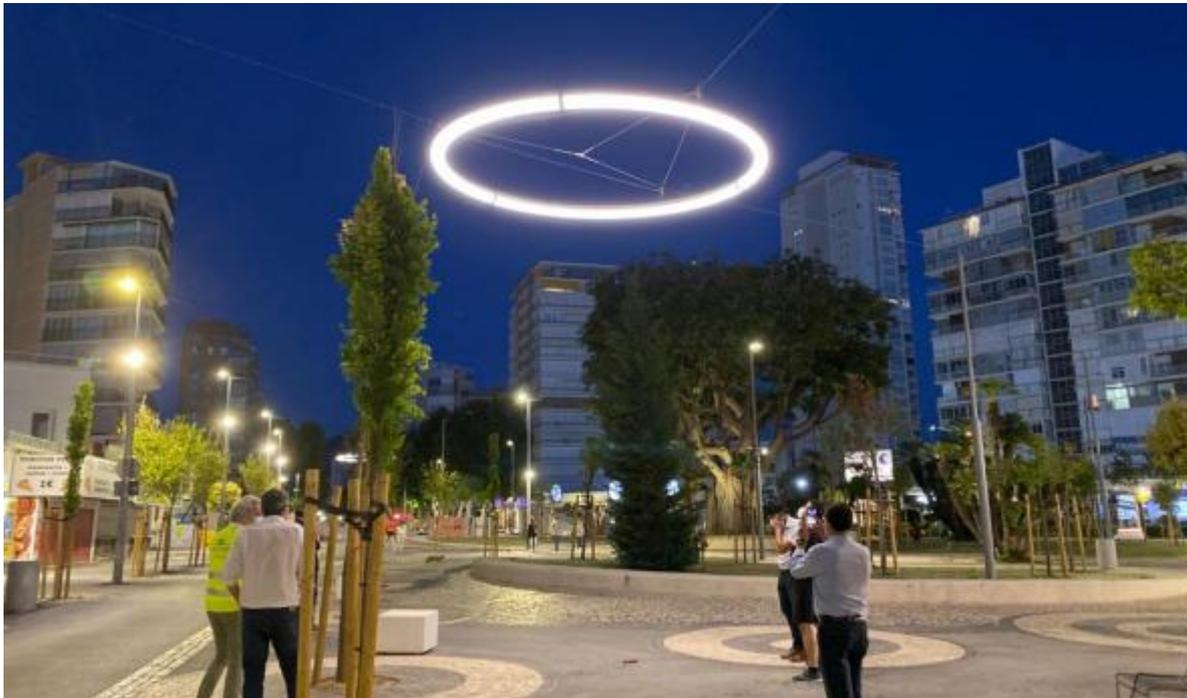
The City Council and the company in charge of the remodeling works on Mediterráneo Avenue have begun the installation of the luminaires proposed in the project, which have been exclusively designed for Benidorm and whose main characteristic is to be suspended by steel cables. Yesterday afternoon, two of the nearly 20 lights planned for La Hispanidad Square were installed, and after the test, the rest are expected to be installed throughout the month of June.
